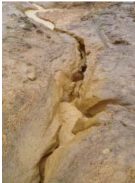
Uncontrolled site erosion by stormwater run-off at the Aotea Block subdivision site, Porirua.
