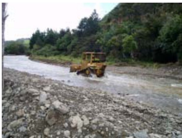
Unconsented stream re-alignment works underway in the Mangaroa Stream, Upper Hutt.
