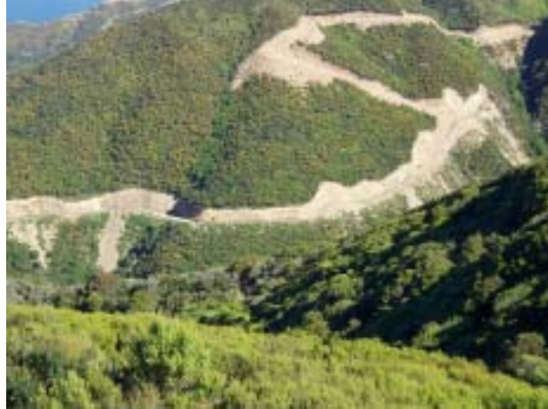
Un-consented track construction above the Carey's Gully landfill site, Wellington.
