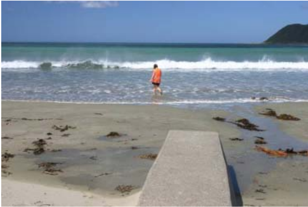
Figure 4.20: Stormwater outfall at Tirangi Road, Lyall Bay.
