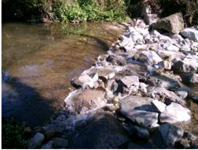
Figure 2.5: Fish pass constructed at the weir downstream of Eastern Hutt Road (left) and a possible barrier to fish passage at the confluence of the Pinehaven Stream with Hulls Creek (right)
