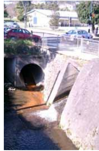
Figure 2.5: Fish pass constructed at the weir downstream of Eastern Hutt Road (left) and a possible barrier to fish passage at the confluence of the Pinehaven Stream with Hulls Creek (right)
