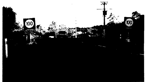
"Works end" sign correctly placed on both sides of the road
