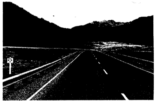
Narrow bridge over Camerons Creek, SI 16, recently widened to improve safety
