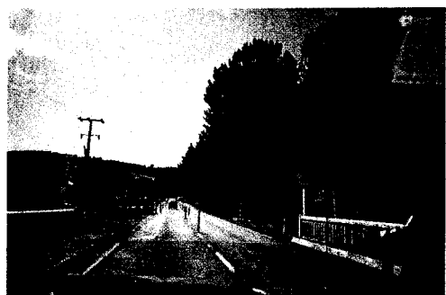
One lane closed due to works, but no temporary speed limit in place
