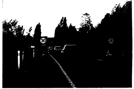
Well placed speed restriction signs on both sides of the road
