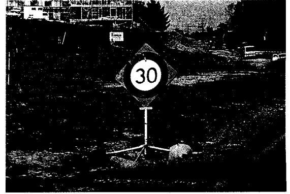
This sign should have a "temporary" plate below the speed limit.
