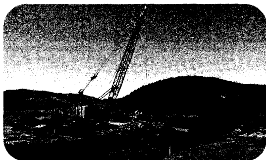
Working on piles at the Pauatahanui Bridge site
