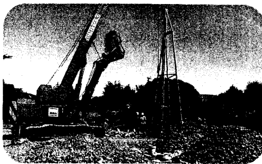
Installing the wick drain on the Pauatahanui Bridge Replacement Project
