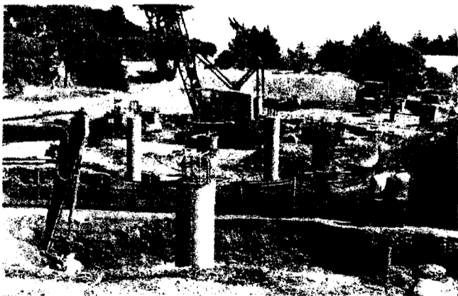
Construction of bridge piles
