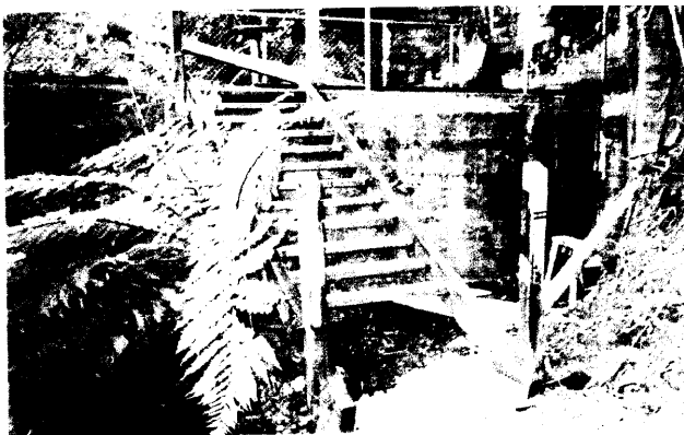
During construction of new ramp, Swingbridge Track, Kaitoke Regional Park.
