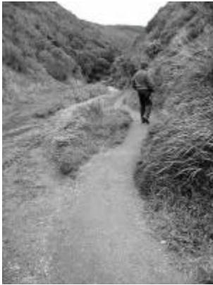
Lower Korokoro track repairs
