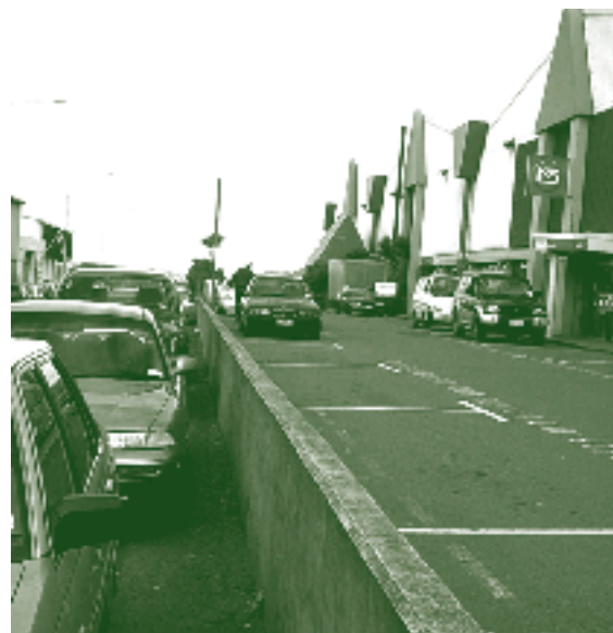
An example of a voluntary action by NZ Post in Petone. You can see by the carpark on the right hand side of the photo that the site has been raised by over 1 metre.
