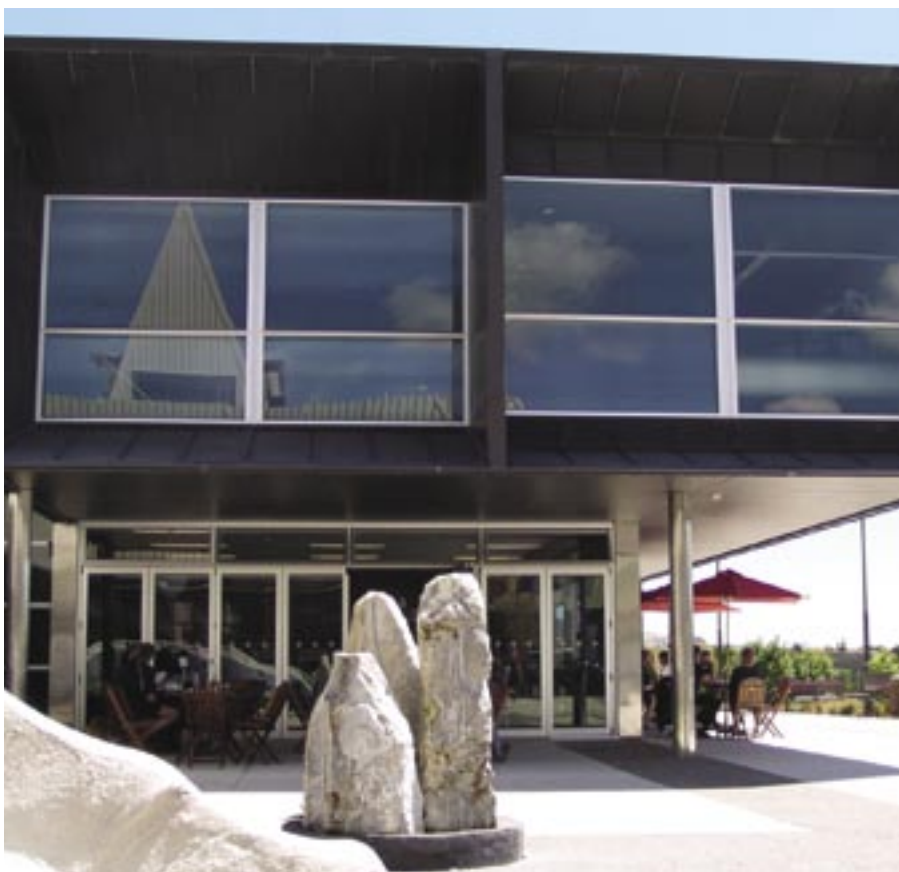
Juken New Zealand timber plant, part of the Wairarapa's Waingawa change area
