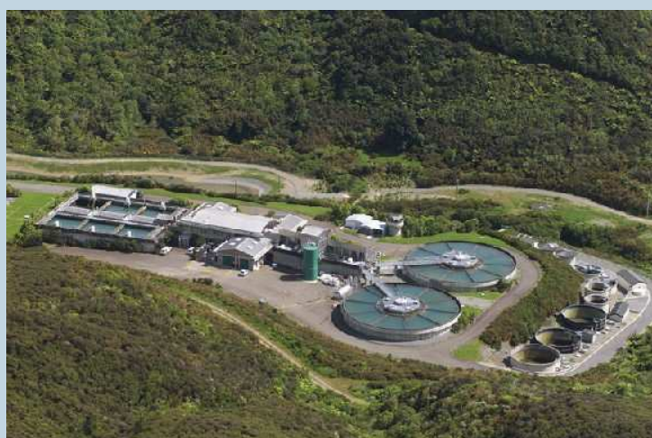
Te Marua Water Treatment Plant
