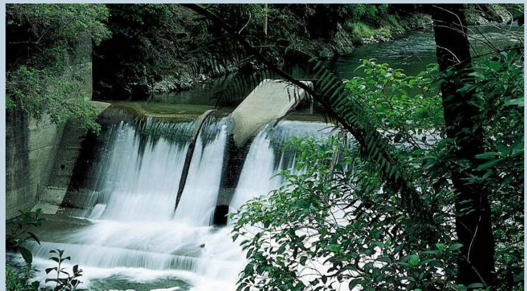
Kaitoke water intake weir
