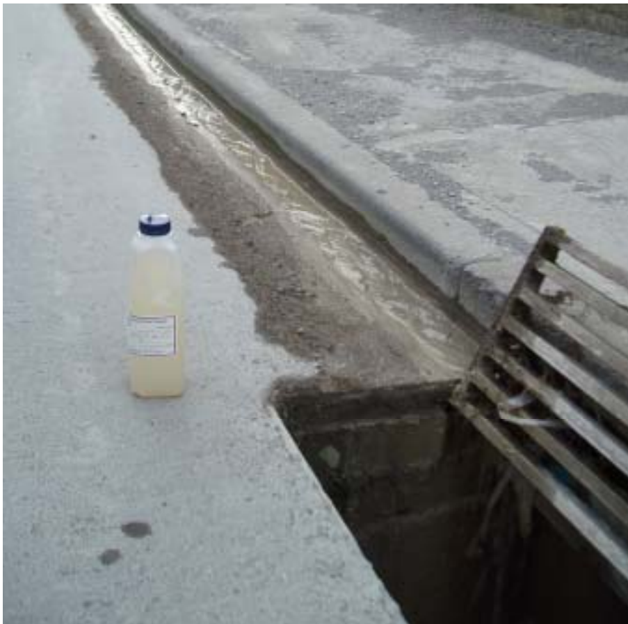
Wastewater runoff from Allied Concrete at Landfill Road
