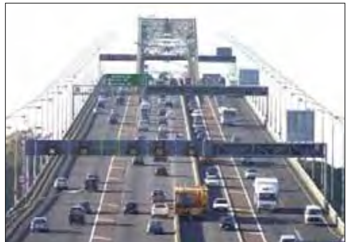
Tidal flow operating on Auckland Harbour Bridge
