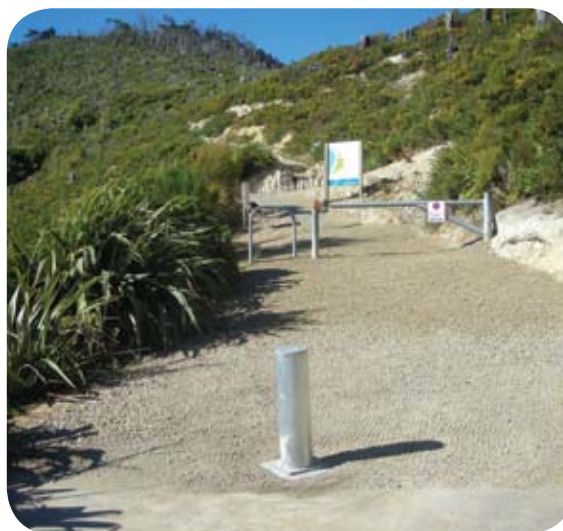
The Ferry Road track was upgraded
