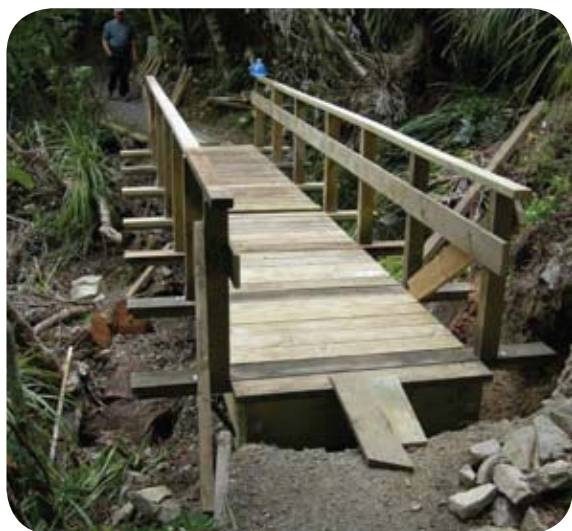
The replacement Mackenzie Track bridge being installed
