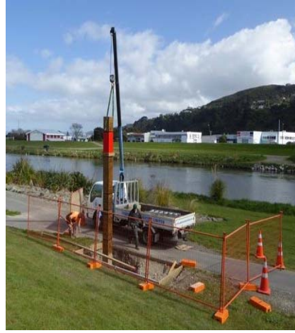
Hutt River Flood Pole Installation
