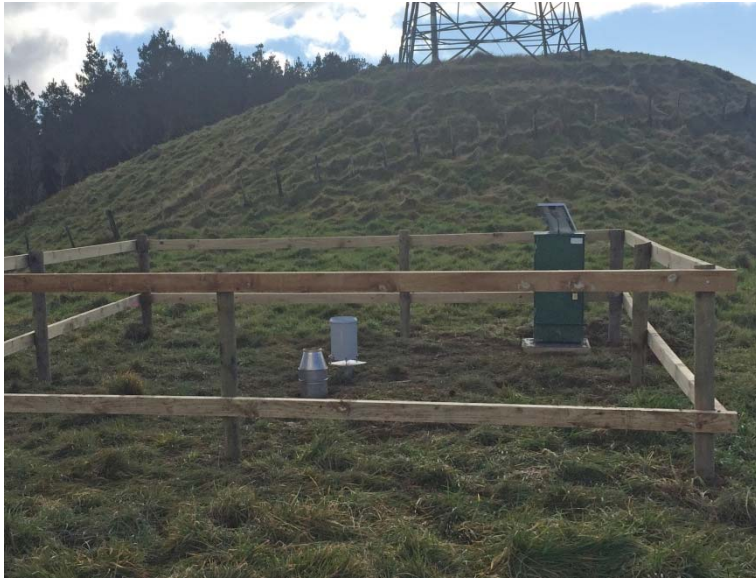
Belmont Trig rain gauge installation
