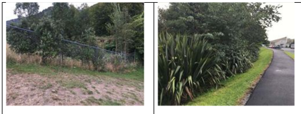
Figure 3 Trees growing in Te Awa Kairangi/Hutt River stopbanks
