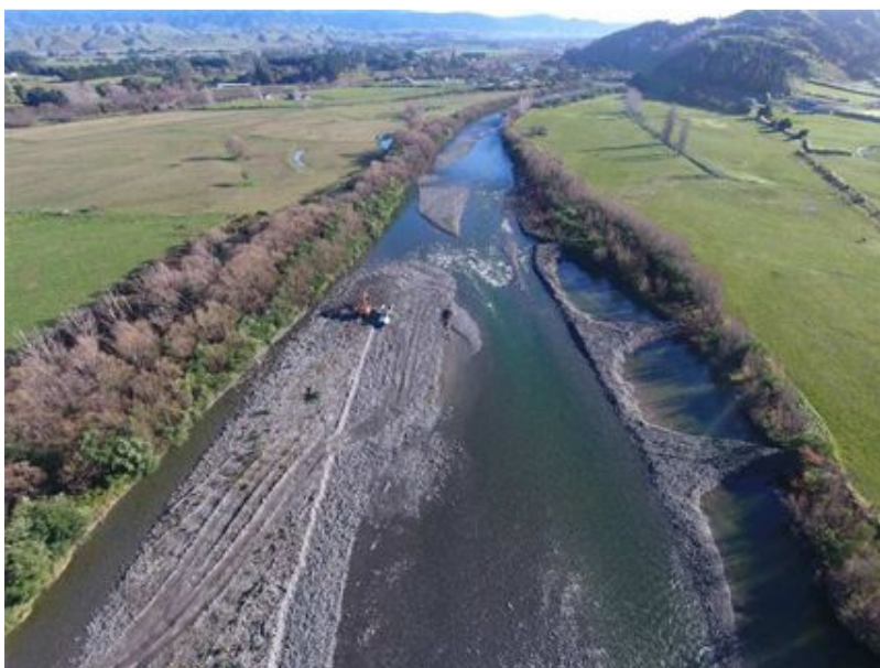
Photo 7: Gravel extraction from problem beach to take pressure off opposite river bank
