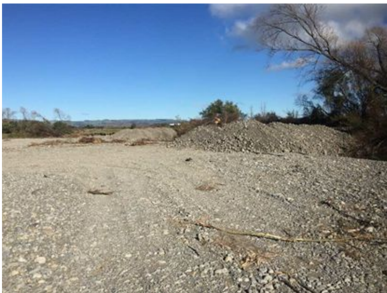
Photo 4: Waingawa River gravel groyne construction
