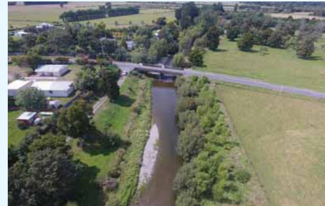
Paierau Road Bridge
