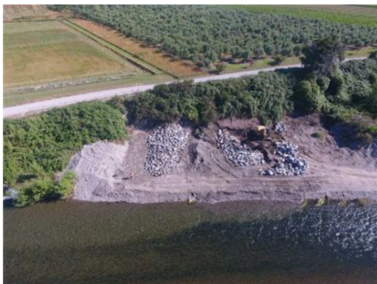
Photo 8: Gladstone reach, Dakins Rd rock groyne construction
