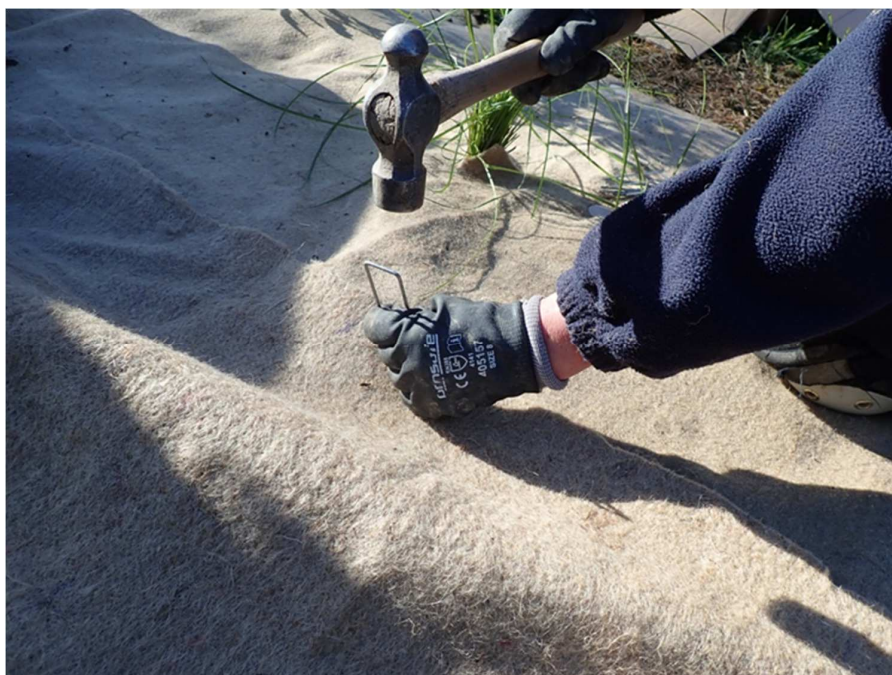
Hammering a steel staple through a join in the EcoJute.
