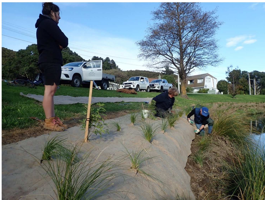
Fitting the second (bottom) layer of EcoJute on the lower slope.
