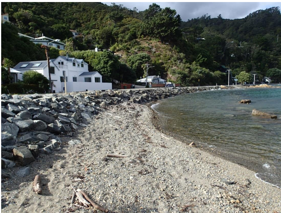
Figure 9-1: Existing revetment to be upgraded, north end of Mahina Bay. The shared path project proposes to upgrade this existing revetment and to extend it seaward to achieve a 5.3 m total revetment width (covering much of the gravel in the foreground). Photo: P5020121, 2016-05-02.
