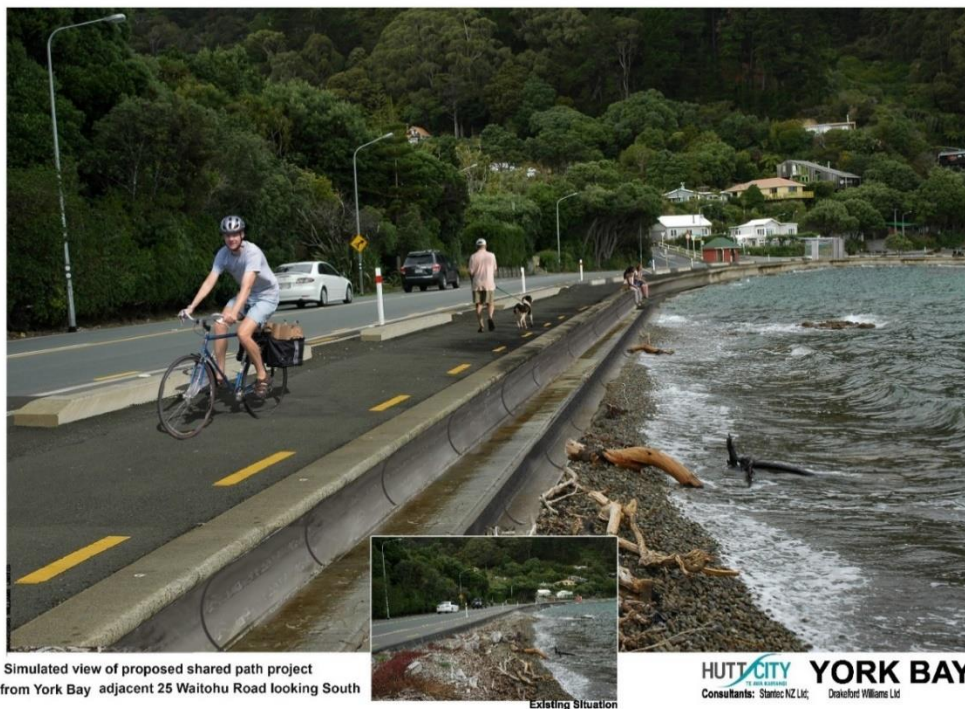
Figure 2-3: Simulated shared path view, northern York Bay, 3.5 m path width, double curve seawall in the foreground and triple curve seawall beyond to Taungata Road. Source: Hutt City Council (2018).
