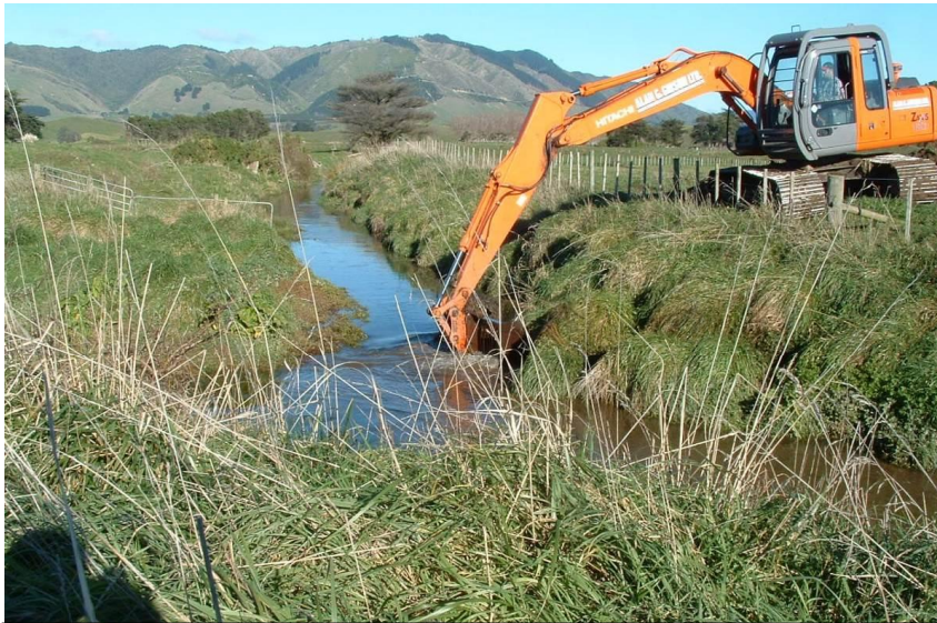
17 Drain clearing (Pahiko Drain)
