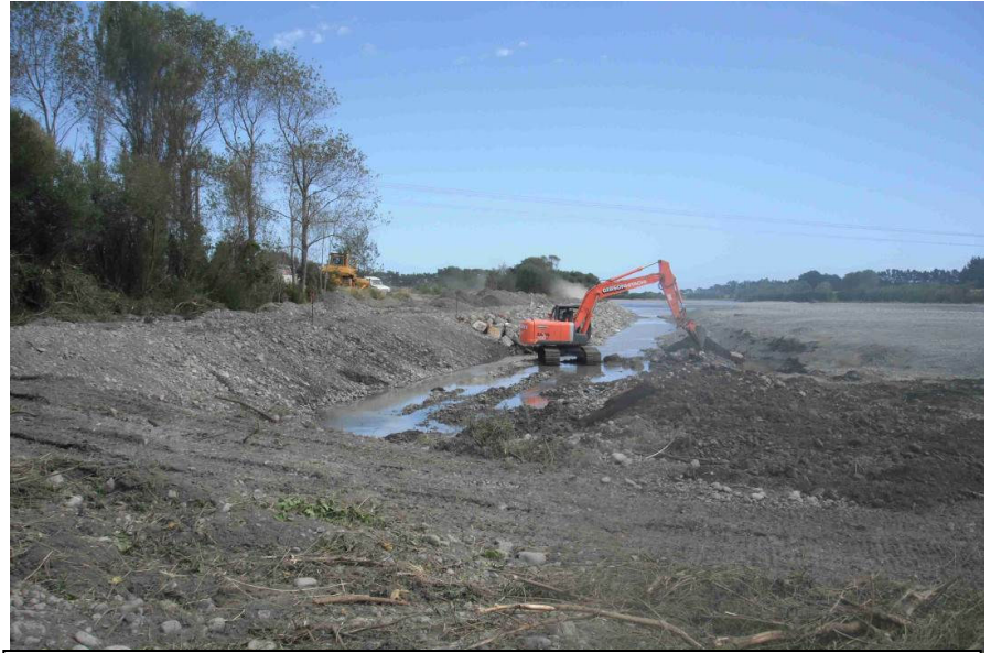
5 Rockline construction (Lethbridge – XS 220 to XS 240 approx)
