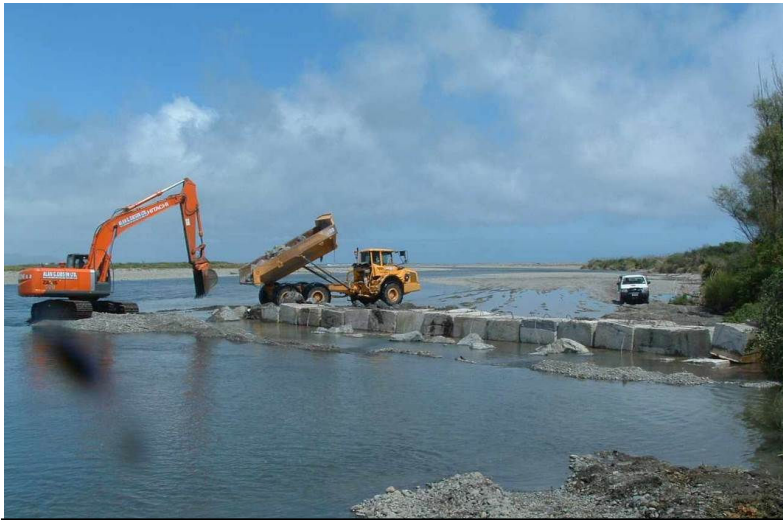
1 Rock groyne construction – placing concrete blocks
