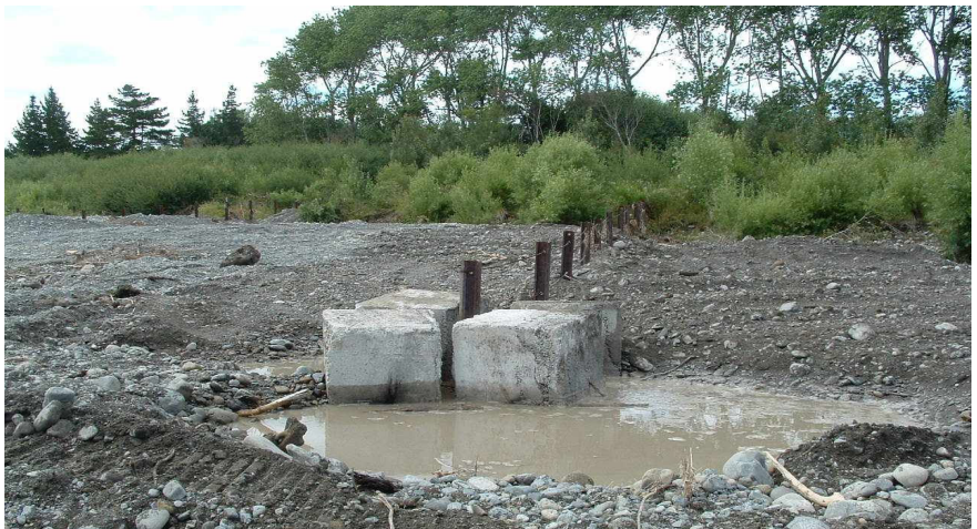
8 Completed debris fence
