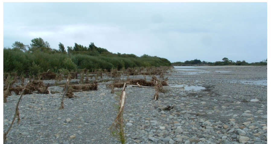
9 Debris fences in operation
