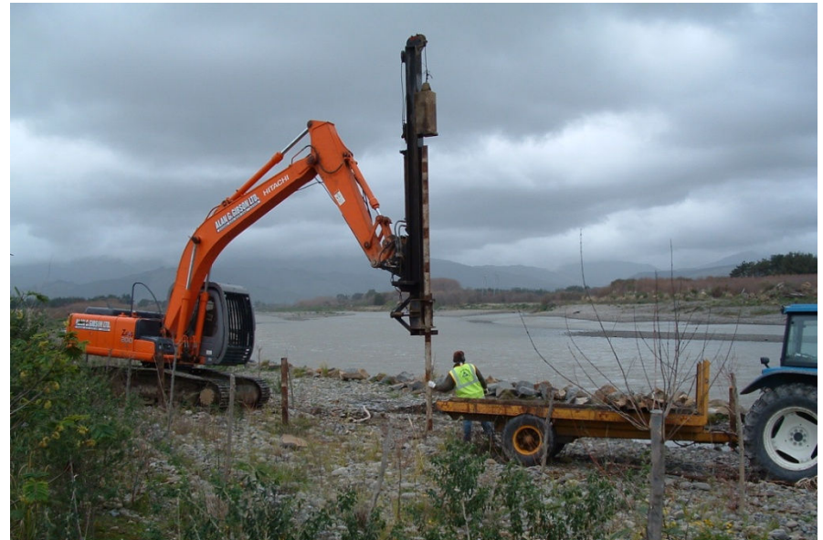
7 Debris Fence construction (driving irons)
