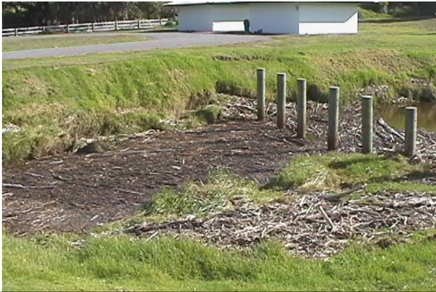
6 Debris arrester (Waimeha Stream)
