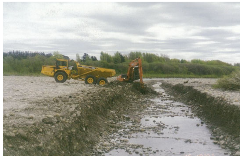
16 Channel diversion cut
