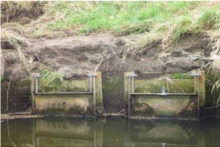
24 Katihiku Drain floodgates
