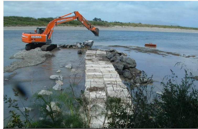
2 Rock groyne construction – placing rock
