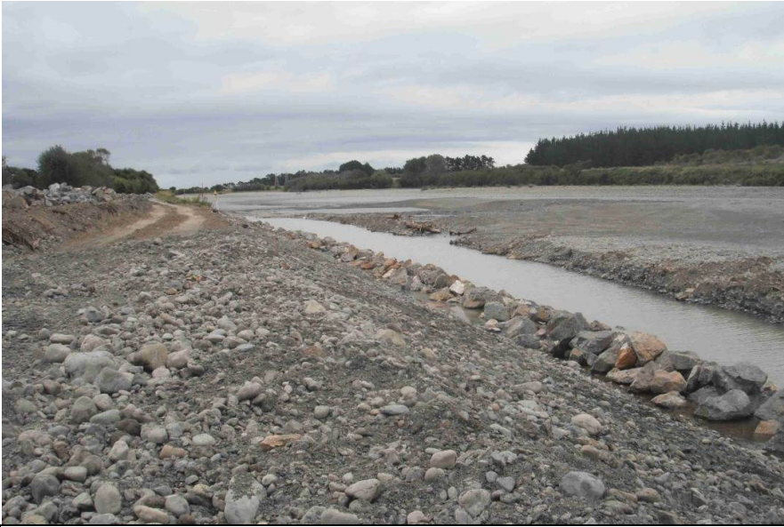
4 Rockline construction (Lethbridge – XS 220 to XS 240 approx)
