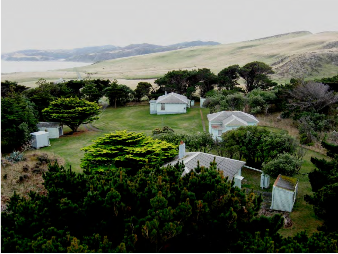
Fig. 8. Keepers' houses and the generator (power) building (centre right) from the south. The garage is at left.
