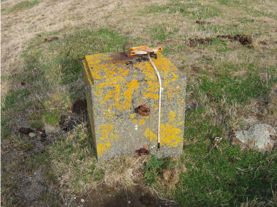
Fig. 18. Concrete counter-weight for the static tensioning stay to the north-eastern mast. It was originally suspended in a steel frame (see Fig. 19).
