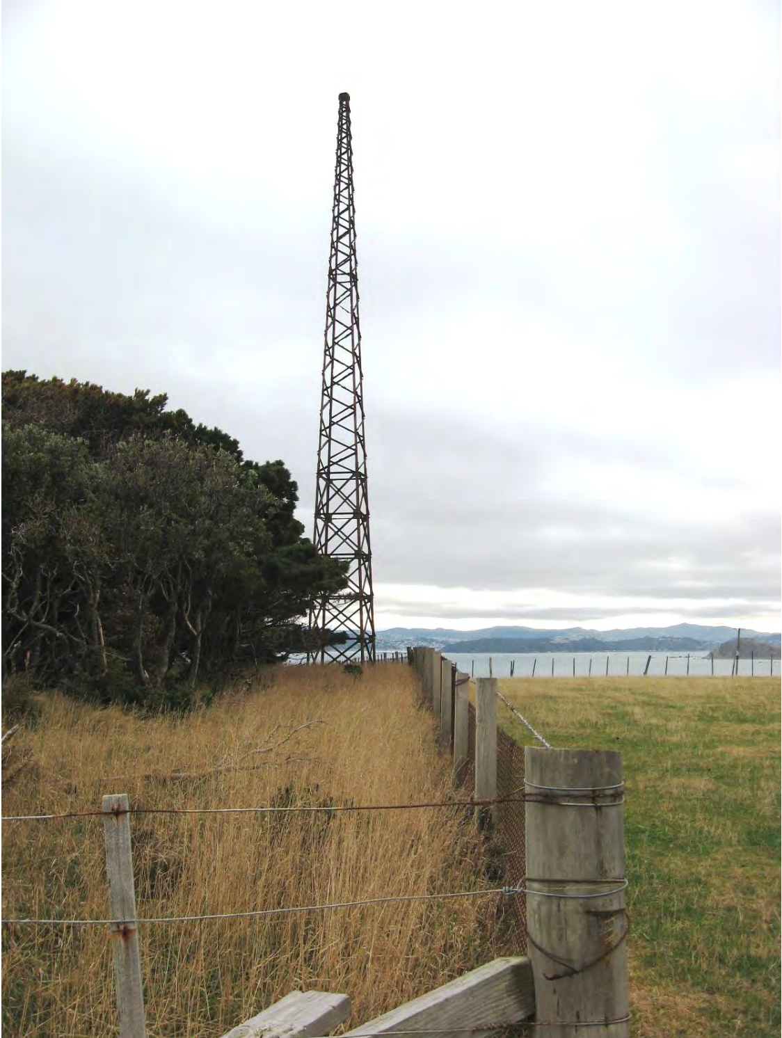
Fig. 16. The north-east aerial mast.
