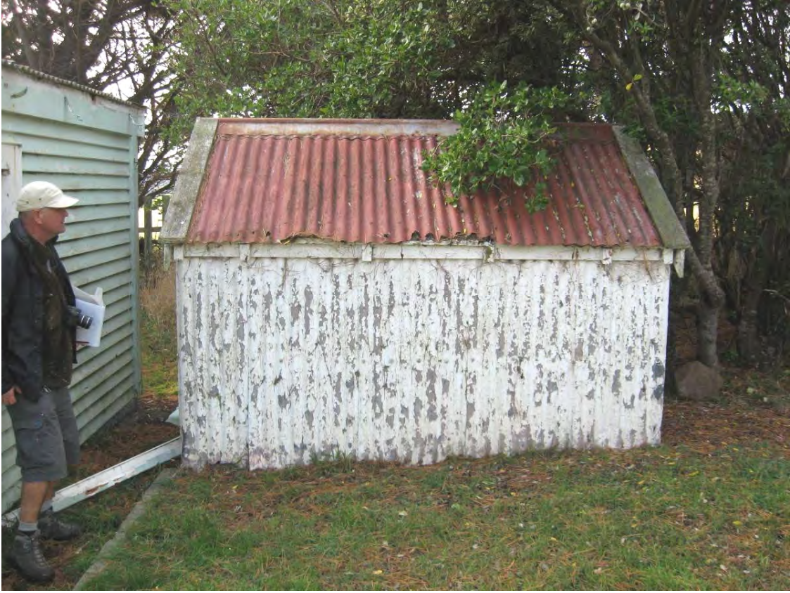
Fig. 11. The Marine Department type store behind keeper's house no. 2.
