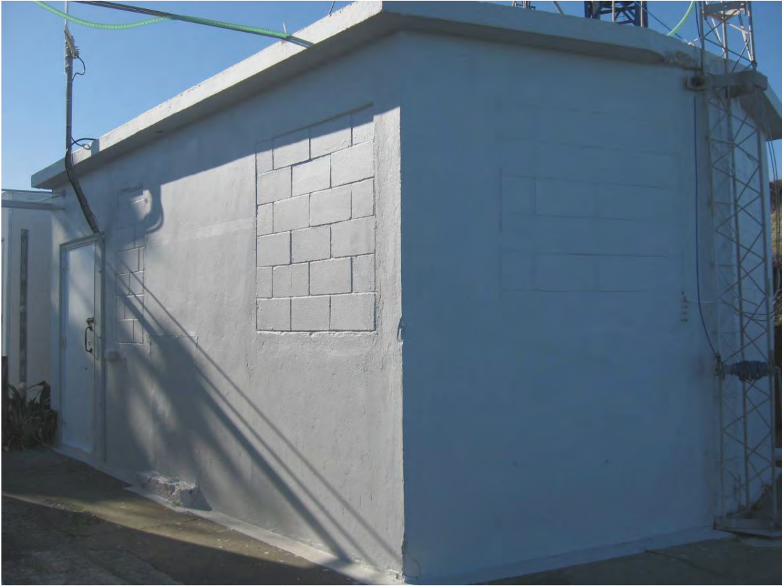
Fig. 23. The WW II radar building from the south-west with the blocked-in bow window and other window apertures.
