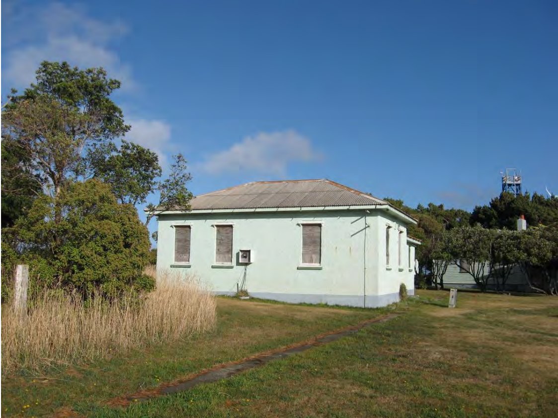
Fig. 13. North elevation of the concrete generator building. Note twin galvanized pipes under the eaves (upper right) which may have held a bracket for the feeder wire to the radio antenna.
