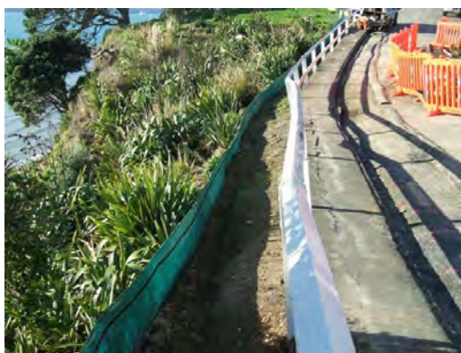
Figure 80: Silt fence installed on edge of works
