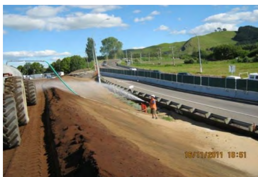
Figure 128: Dust suppression using soil binders/polymers
