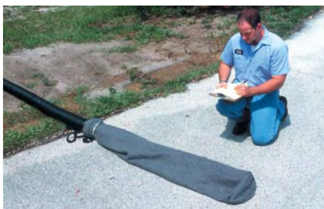
Figure 106: Dewatering bag and pipe sock
