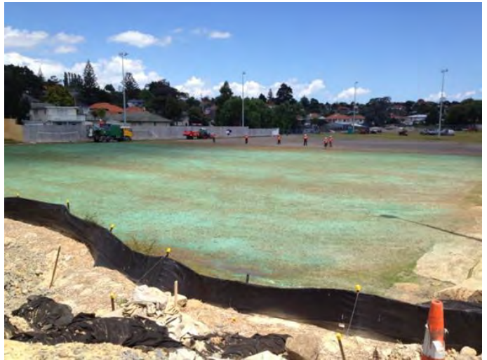
Figure 49: Sports field being hydroseeded. Sediment control remains installed until an 80% grass strike has established
