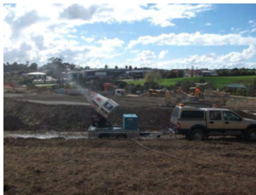
Figure 127: Snow blowing machine to provide dust control during a liming operation
