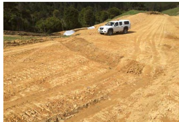
Figure 23: Contour drain installed across access track
