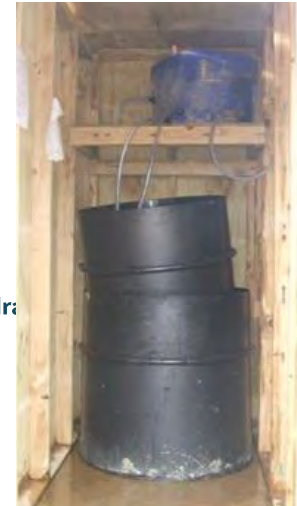
Figure 104: Flocculation shed
