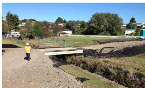
Figure 114: A temporary bridge in the process of being installed
