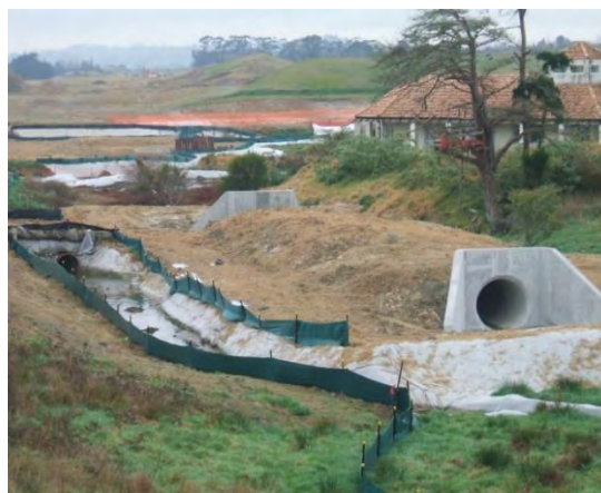
Figure 118: Examples of temporary stream diversion installed to allow permanent culverts to be installed off-line
