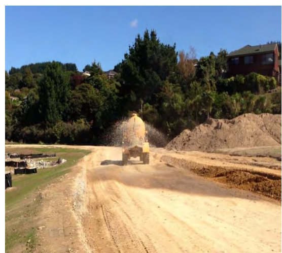
Figure 126: Dust suppression using a water cart
