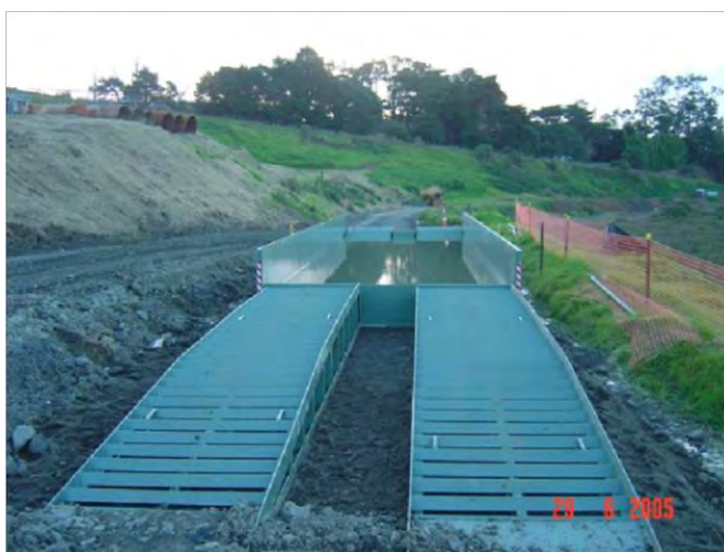
Figure 38: Example of a shaker ramp
