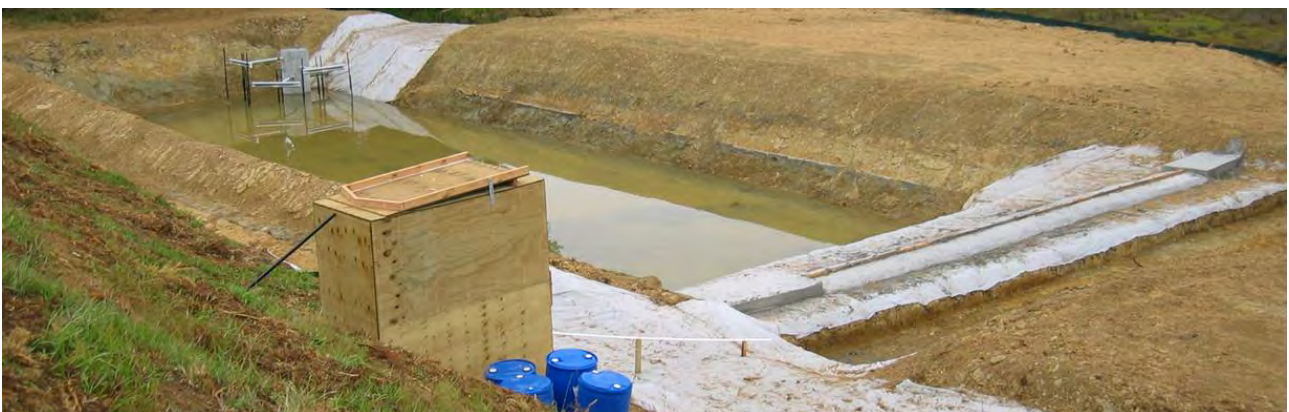
Figure 10: A typical earthworks construction site
