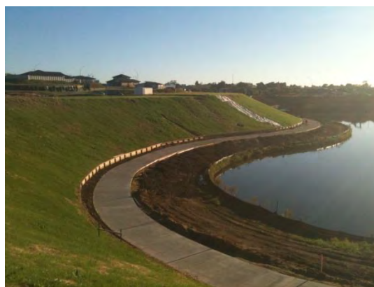
Figure 43: Grass stabilised earthworks site. Batter and building platforms
