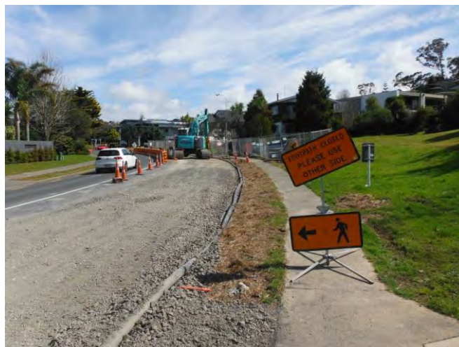
Figure 110: Use of stabilisation products and progressive stabilisation
