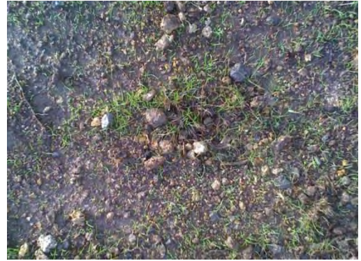
Figure 44: Initial grass strike - not stabilised
