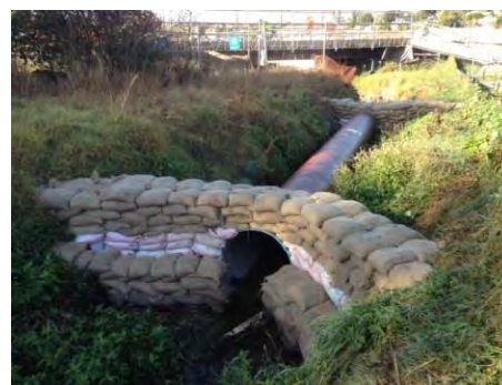
Figure 115: In the process of constructing a temporary crossing
