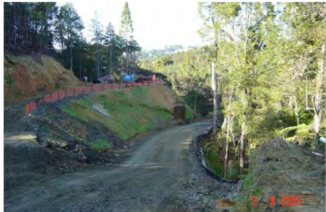
Figure 11: Northern Motorway construction site - minimising disturbance
