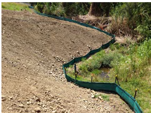
Figure 85: Contours create the same effect as returns in this case
