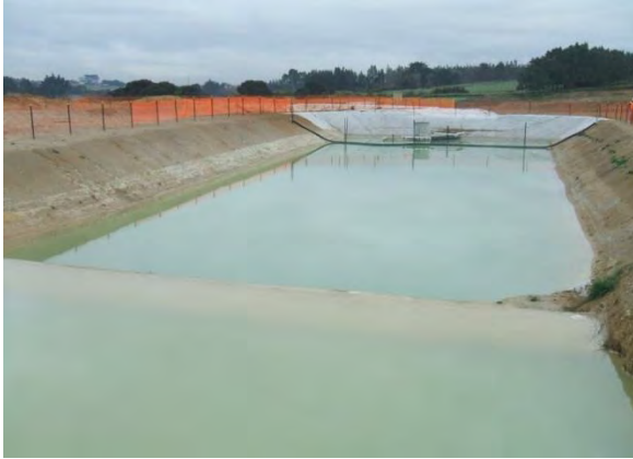
Figure 76: Level spreader across the full width of the pond
