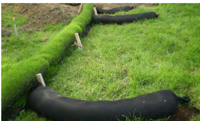
Figure 91: Compost silt socks with returns installed
