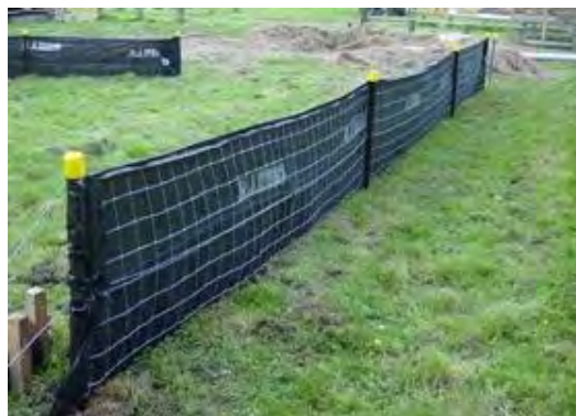
Figure 87: Super silt fence
