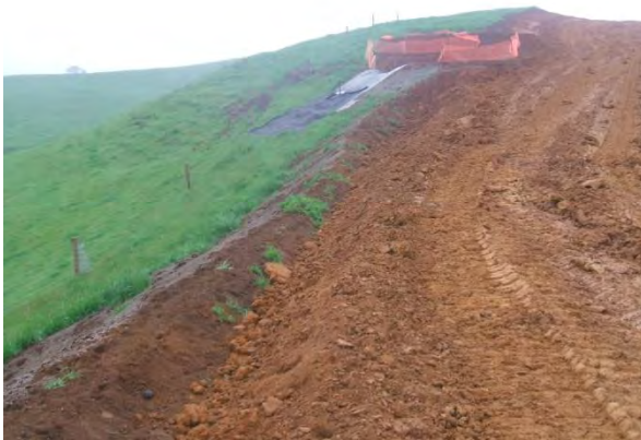
Figure 124: Decanting earth bund and diversion bund installed during a farm track construction
