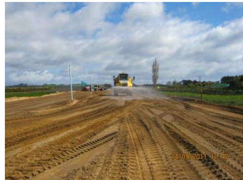
Figure 129: Water truck dampening down the works area
