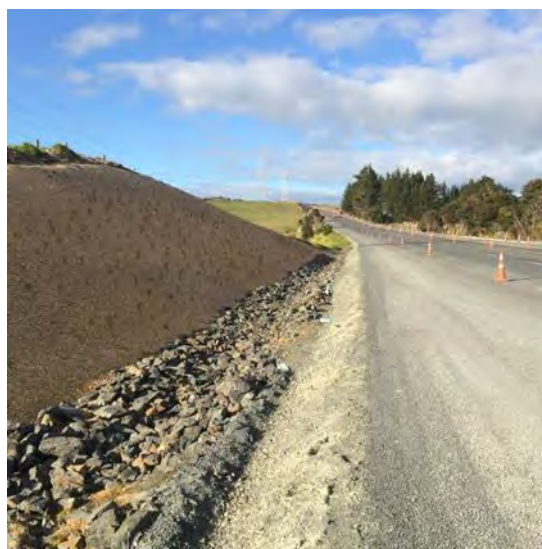
Figure 57: Woodchip to stabilise the finished batter slope
