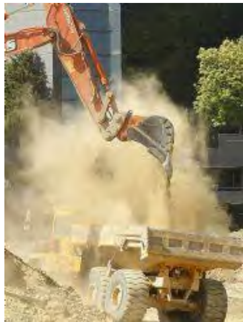
Figure 125: Forward planning and management to minimise dust provide the best options for control
