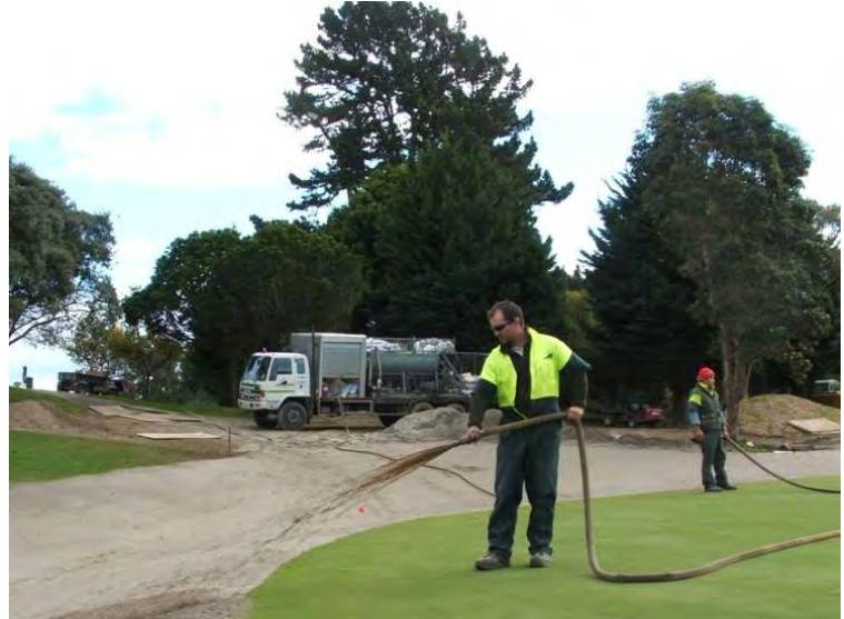
Figure 48: Specialist application of hydroseed
