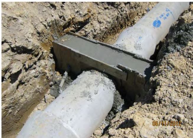
Figure 71: Example of an anti-seep collar
