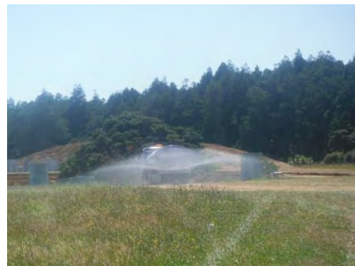
Figure 130: Regular wetting of the haul road
