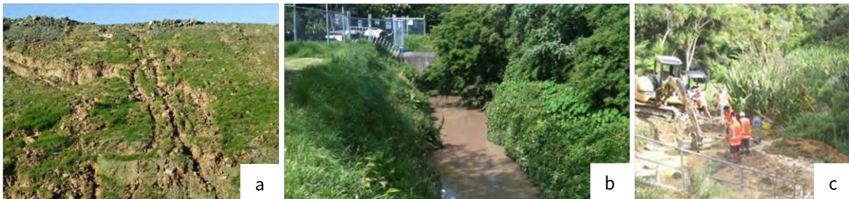
Figure 3: Examples of erosion (a) and sediment discharge (b and c)
