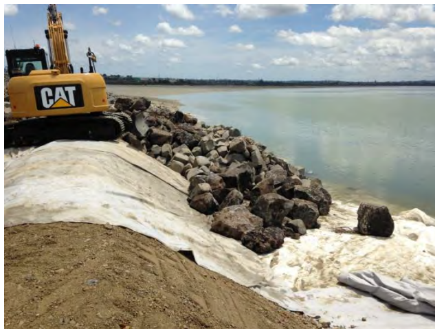
Figure 134: Use of geotextiles and coastal protection rock (SouthernSkies, 2018)
