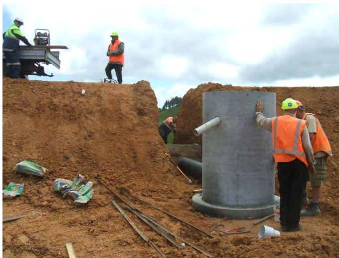
Figure 75: Installation of the outlet pipe and the anti-seep collars
