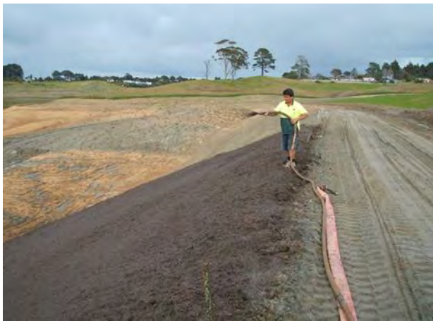
Figure 55: Hydromulch application
