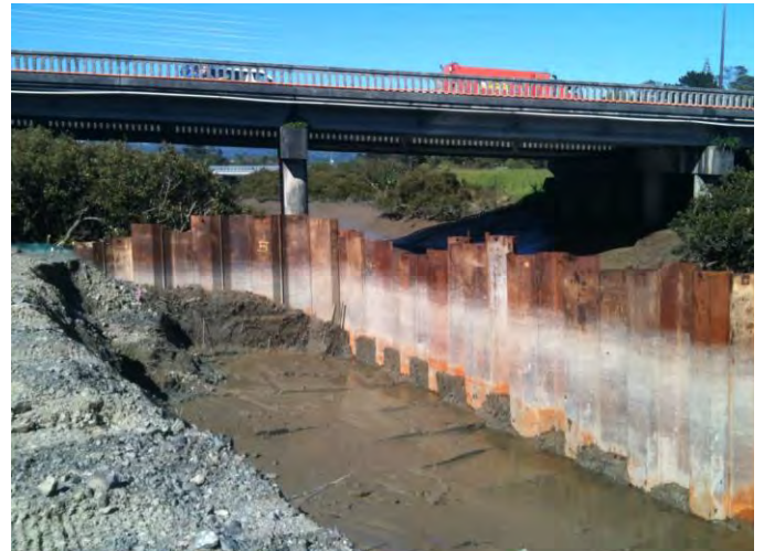
Figure 132: Sheet pile coffer dam (SouthernSkies, 2018)
