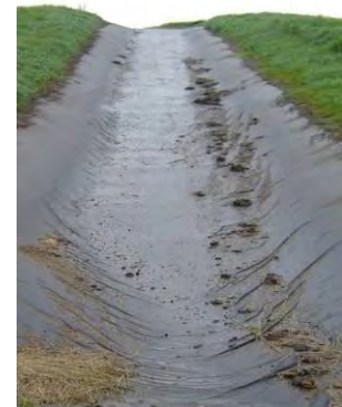
Figure 31: Geotextile lined flume
