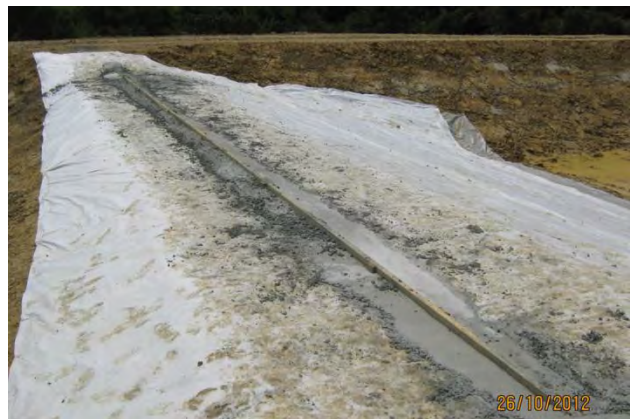
Figure 69: Example of a level spreader
