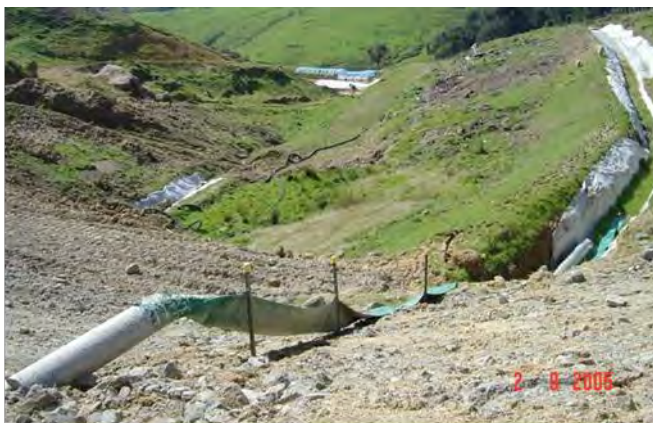
Figure 12: Flume installed to protect steep slope
