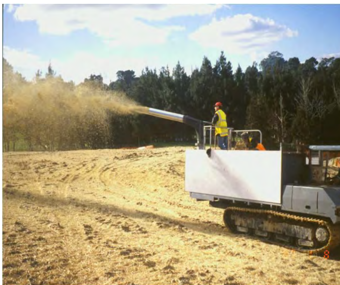
Figure 54: Specialist application of hay mulch
