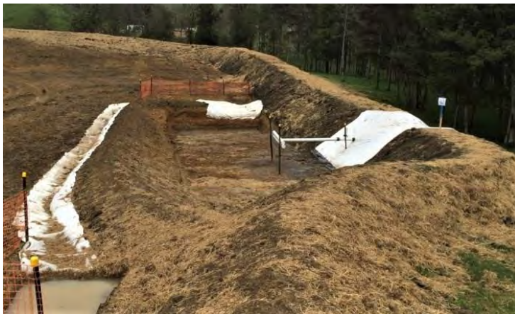
Figure 78: Decanting earth bund system and close up of T-bar dewatering device.
