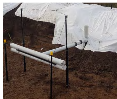
Figure 78: Decanting earth bund system and close up of T-bar dewatering device.
