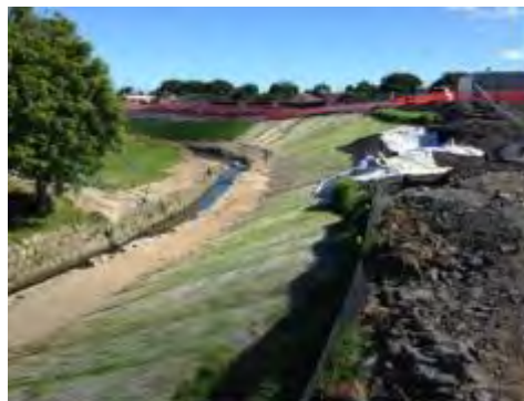
Figure 63: Coconut fibre blanket used to stabilise batters while allowing grass to grow through
