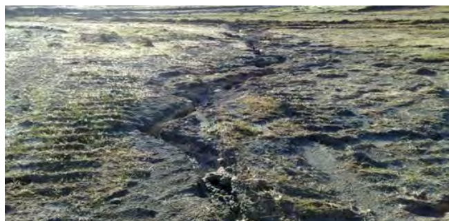
Figure 47: Loss of topsoil and grass seed after heavy rain event. Will require stabilisation and reapplication
