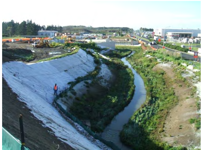
Figure 58: Geotextile used to temporarily stabilise the batter face
