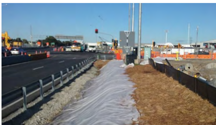
Figure 109: Progressive stabilisation in limited space
