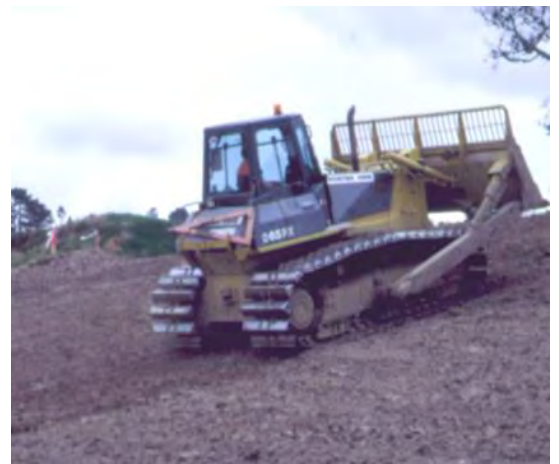
Figure 39: Surface roughening with bulldozer
