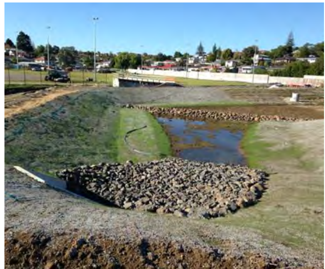
Figure 50: Recently applied hydroseed on a stormwater wetland
