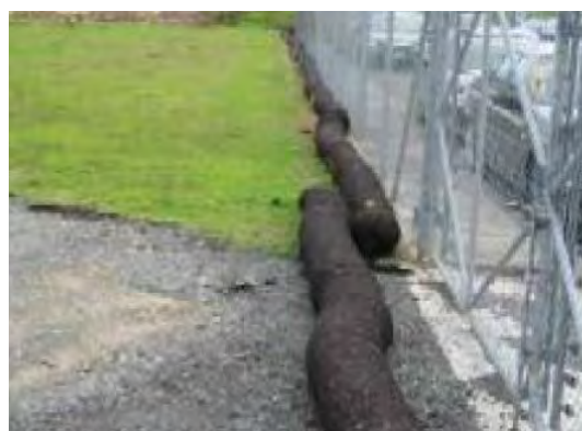
Figure 92: Silt sock with 1 m overlapping joint
