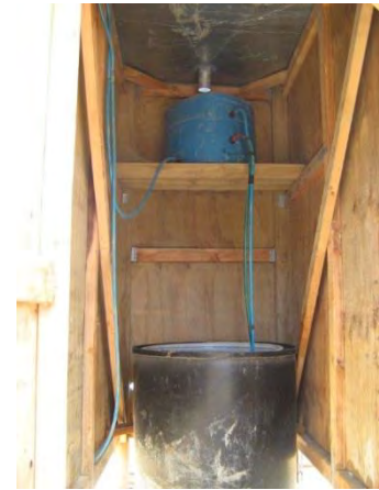
Figure 103: Header tank
