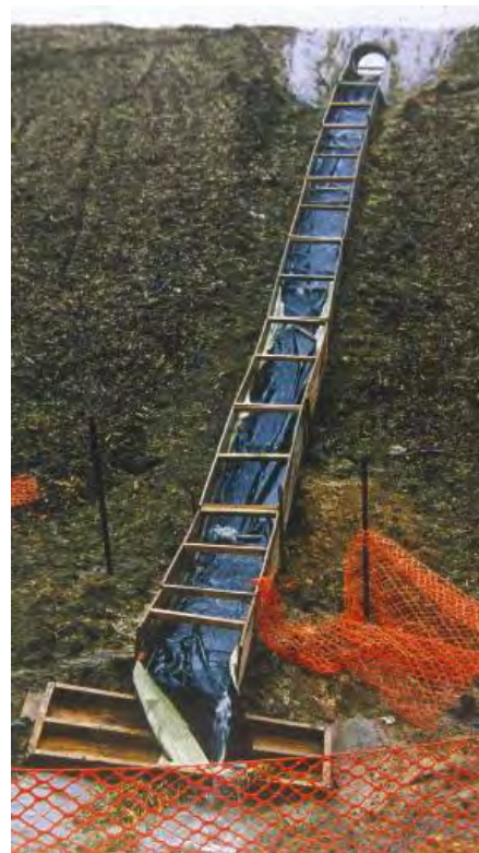
Figure 32: Wooden flume lined with impervious material
