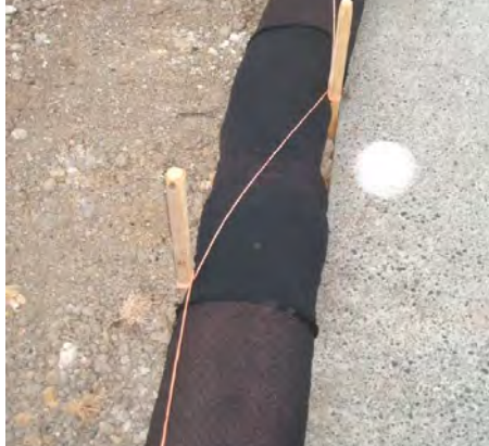
Figure 93: Silt sock joined using a sleeve and pegged and secured using baling twine with 1 m overlapping joint
