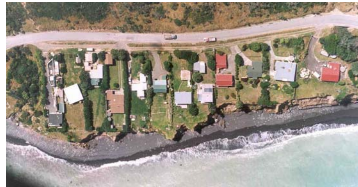
This photograph, taken in February 2000, shows houses under threat at Whatarangi. Several buildings have been lost to the sea in this area. Over 10 metres were lost between 1996 and 2001.
