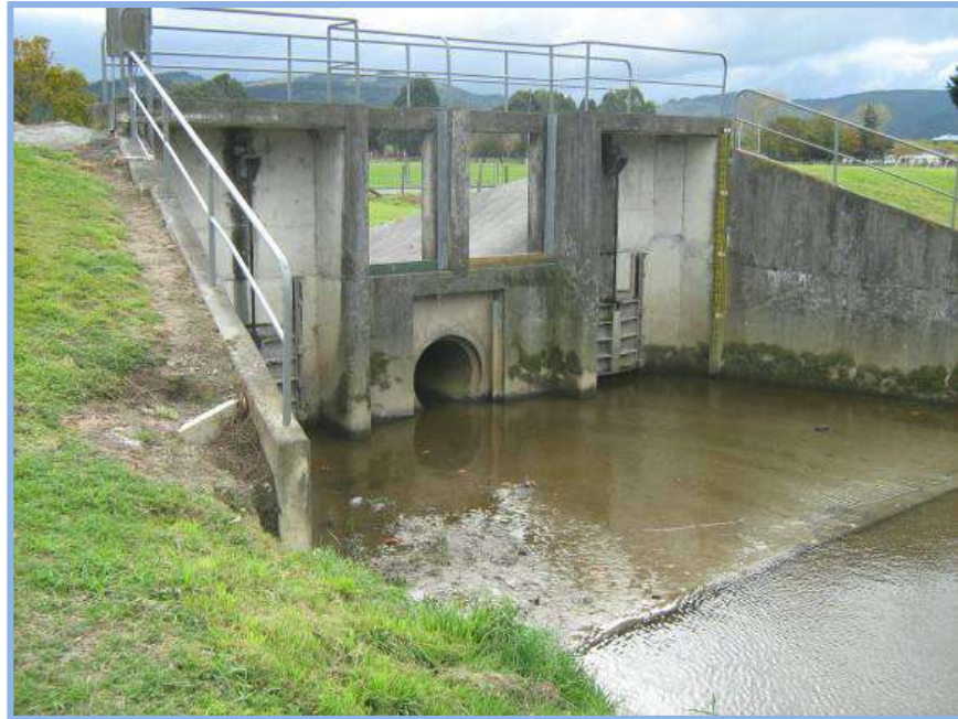
■ Figure 9 Hulls Creek Detention Dam
