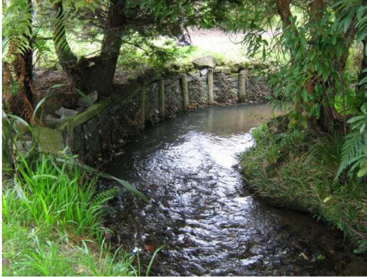
Location F. Gabion retention.
