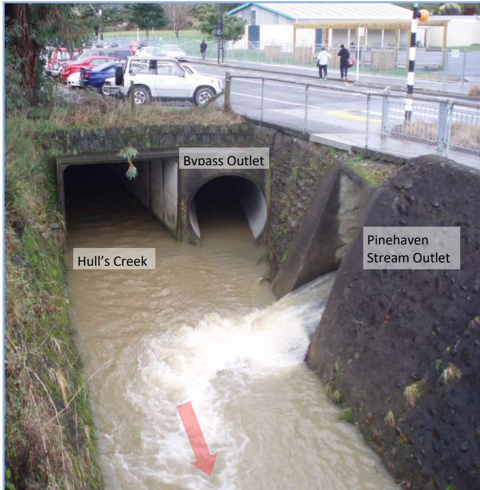
■ Figure 35 Outlets of the Bypass and the Pinehaven Stream
