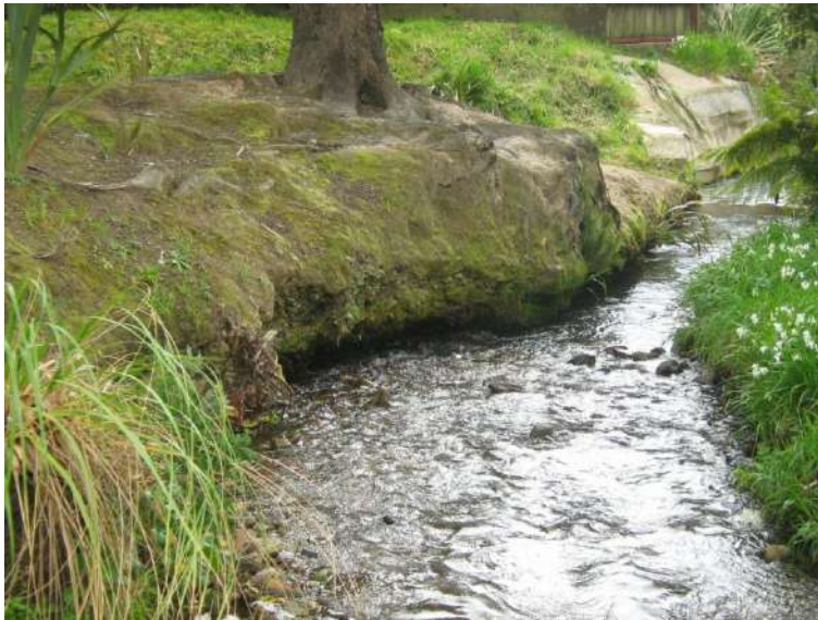
Location C. Undercutting of bank.
