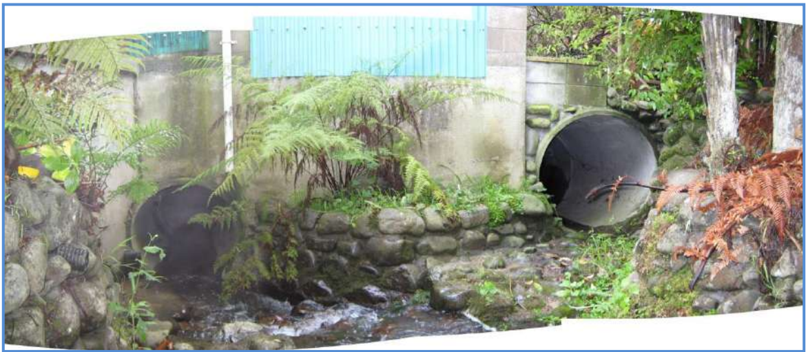
■ Figure 24 Twin culverts under driveway and garage of 47 Elmslie Road
