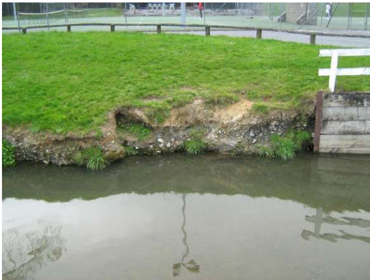
Location A. Eastern Bank downstream of culvert
