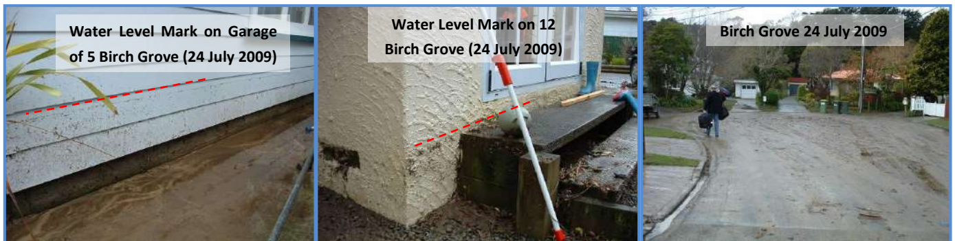
■ Figure 29 Flooding recorded in Birch Grove following the 23 July 2009 Storm
