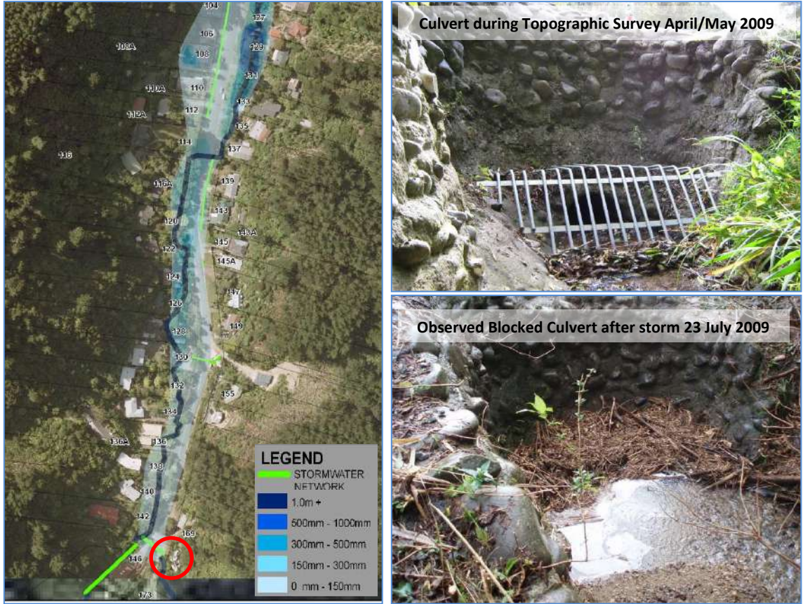
■ Figure 20 Predicted 100 year flood extents at the top end of Pinehaven Road
