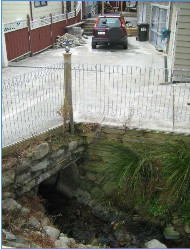
■ Figure 25 Culvert under 19 Forest Road driveway and predicted flooding in a 10 year flooding event.
