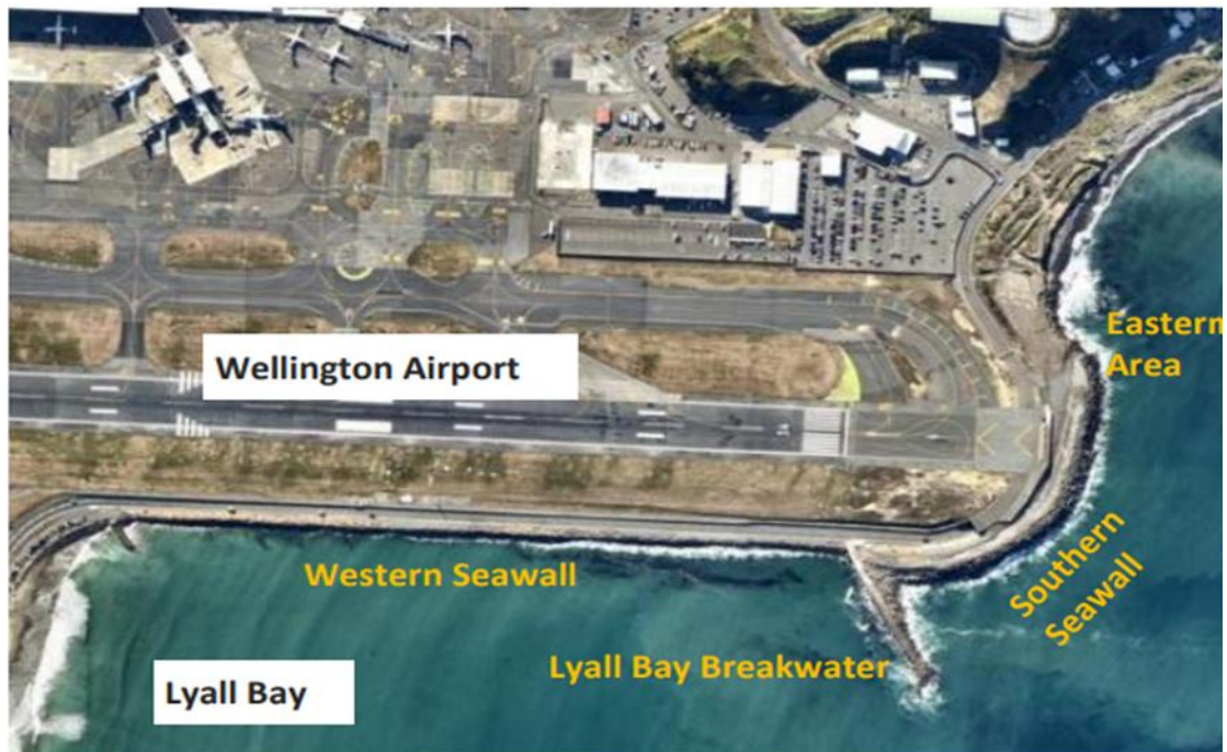
Figure 2: Seawall Structures Lyall Bay
