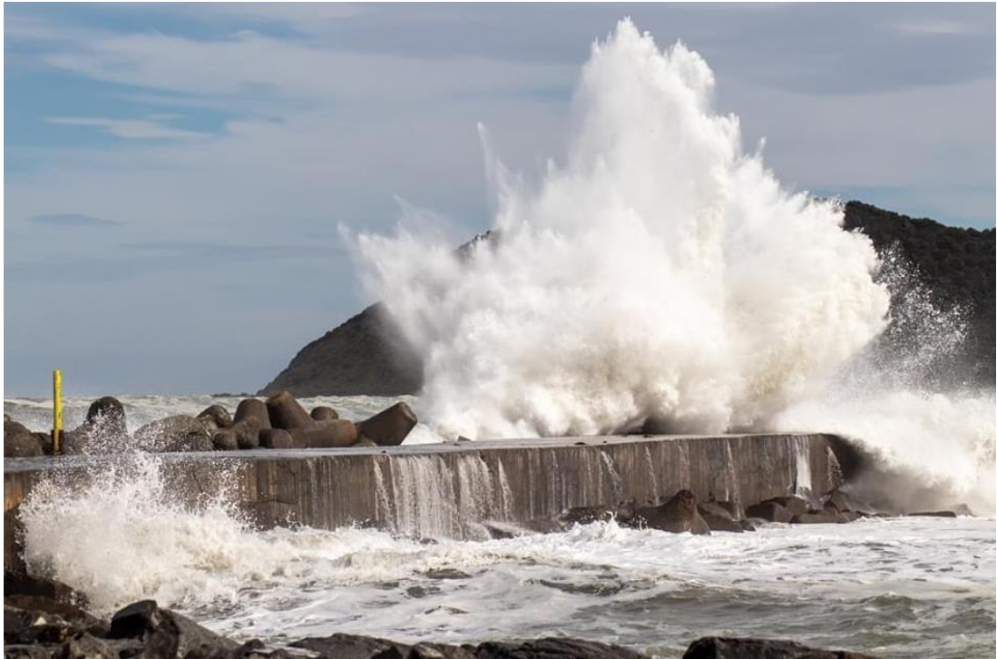
Photo 6: Lyall Bay Breakwater
