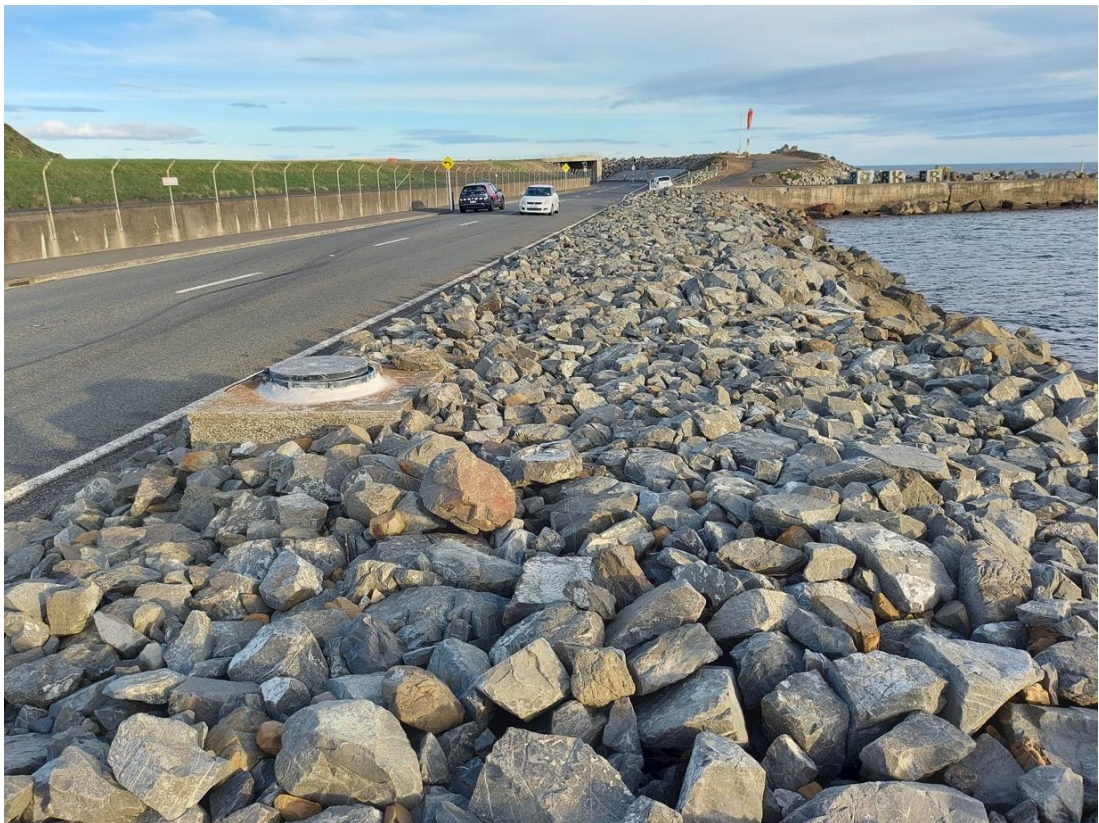
Photo 7: Moa Point Road – crest of western seawall.
