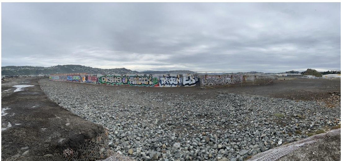
Photo 3: Wave trap and gabion basket wall - looking from Moa Point end of Southern Seawall towards the west.
