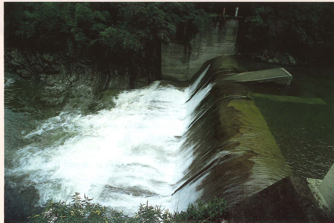
Kaitoke Weir, showing the intake structure at right.
