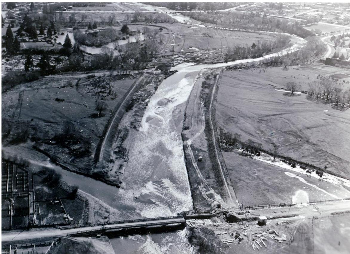
Figure 2.2: View upstream from previous Colombo Road bridge (additional spans under construction, ca. 1935)
